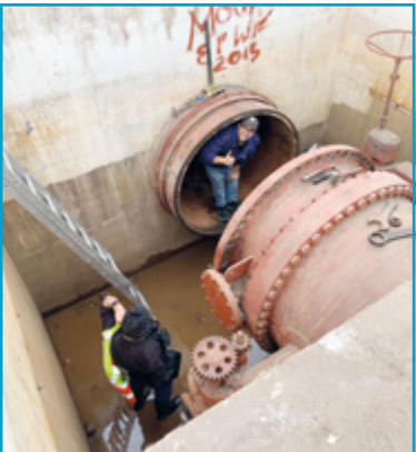
Waterworks: City Water and Sanitation team members worked round the clock for three days to complete essential maintenance and valve replacements on the Cape Flats bulk water pipeline in September.
